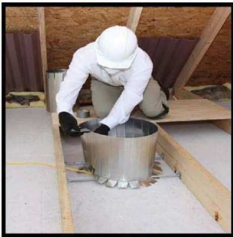
Building a barrier to protect non-IC rated lighting
