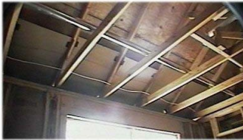
Cardboard baffles installed in attic with pre-built truss construction
