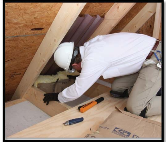
Snugly insert fiberglass into the eave by hand.
