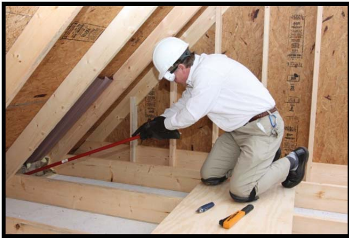
Use a broom to make sure fiberglass is snug if access to eave is difficult.
