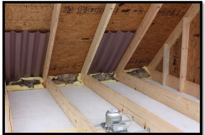
Polyvents were used because of the stick built joist system in this attic. Vents and blocking are in place. Now we're ready to move on to building a barrier for our recessed light!
