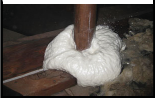
Foam used to seal plumbing bulkhead
