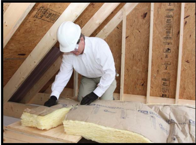
Cut strips of fiberglass sized to prevent loose TAP from entering the eave.
