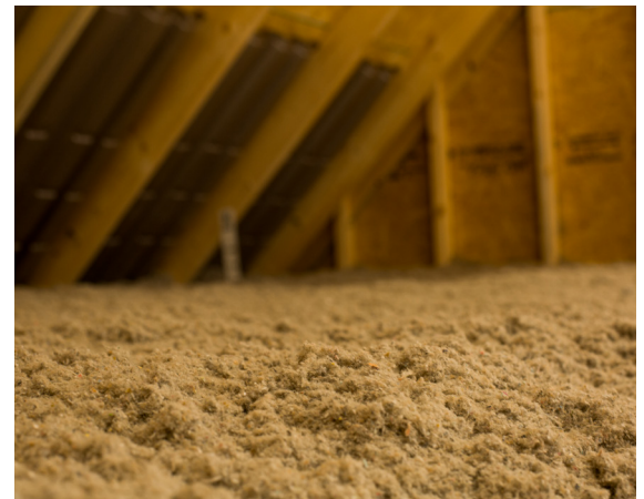
A Completed T·A·P® Attic Job
